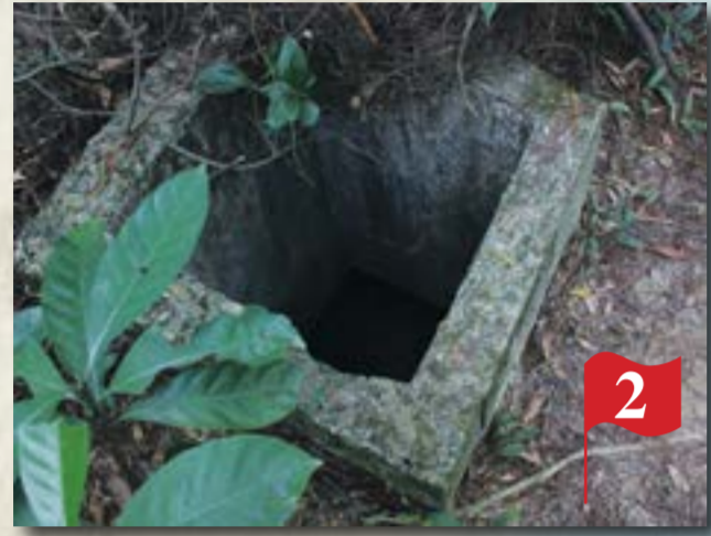
▶ 隧道通風口 Air vent of the tunnel
